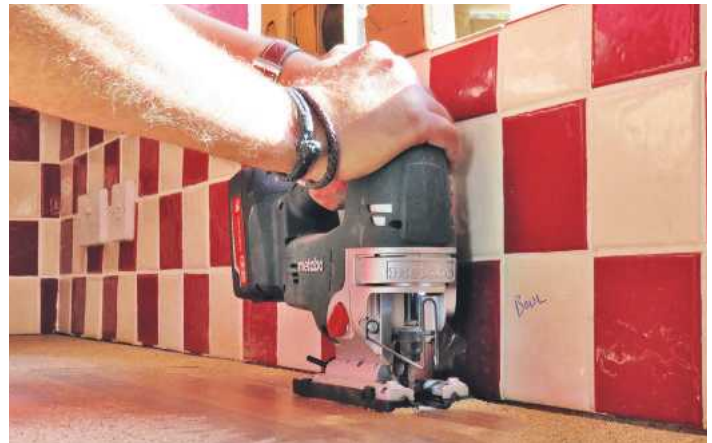
▲ You can also work tight to walls with tops in situ
